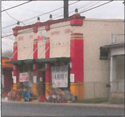
Commercial Building 105 S. Zarzamora
