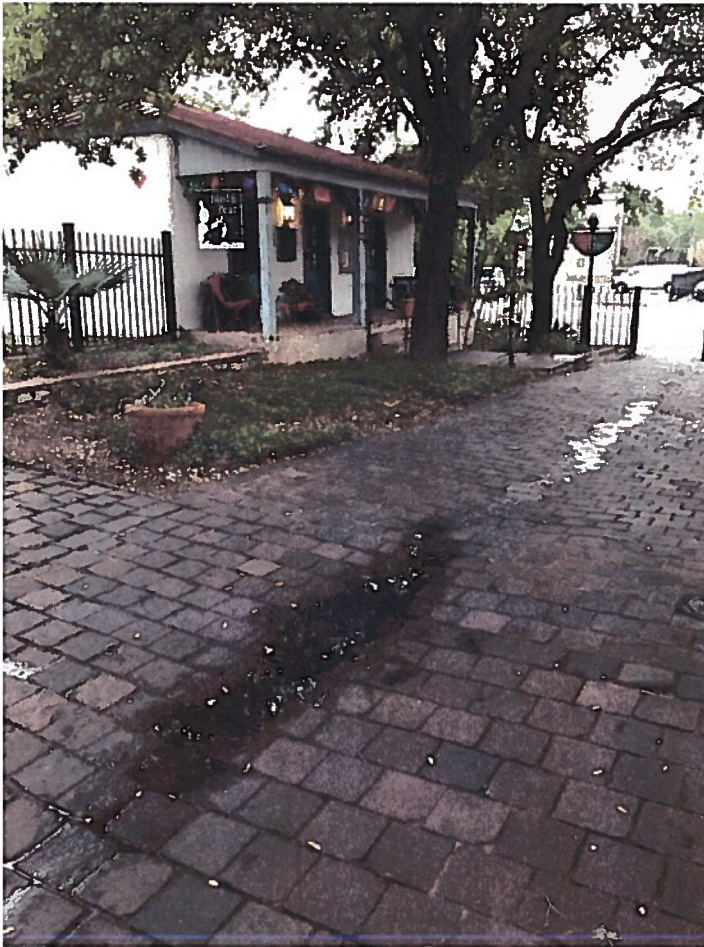
Figure 23. Poor drainage conditions on King Philip V Street.
